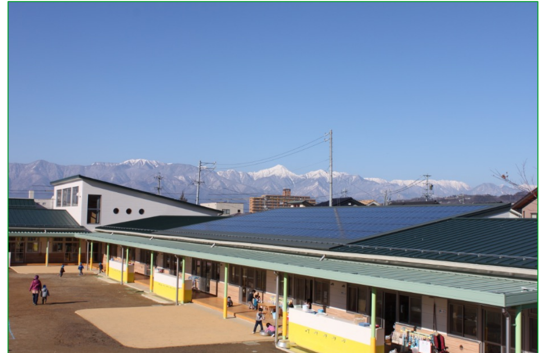
Solar power generation equipment is to be installed sequentially.
